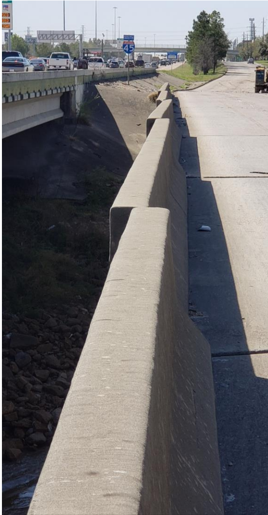
I45 SOUTH BOUND SERVICE ROAD (EAST BARRIER)
